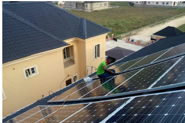
Solar Panel Installation on Homes
