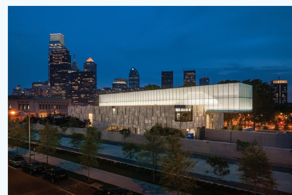
The Barnes Foundation / Tod Williams + Billie Tsien © The Barnes Foundation
